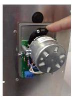
Move the adjustable cam to the right to adjust the minimum position. Make sure to re-tighten the cam locking screw and power damper open and close in order to check position setting.
