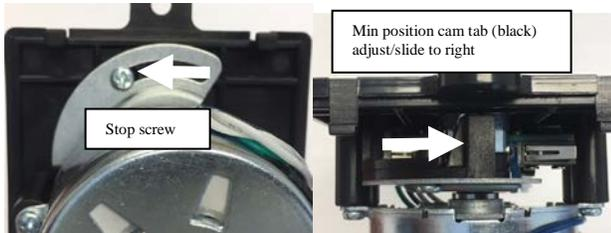
Move the adjustable cam (black section of cam) to the right to adjust the minimum position. Make sure to re-tighten the cam locking screw and power damper open and close in order to check position setting. Reattach the actuator cover.
